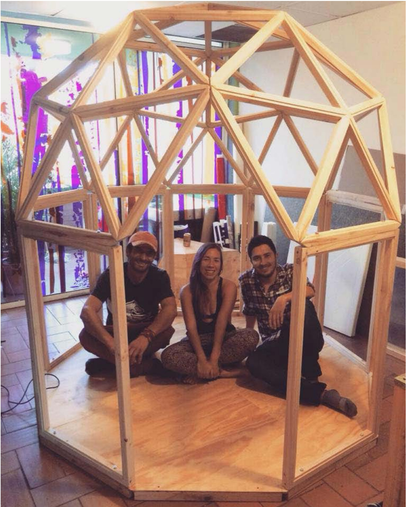
Finished dismountable structure made of pine wood. Location: Angelica's studio. Sebastian Monsalve, architect and Juan Camilo Ortega, builder
